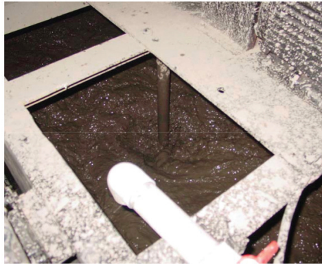
Raw dredged material of about 35 percent solids is being diluted in the mixing tank to about 12 percent solids prior to treatment.
